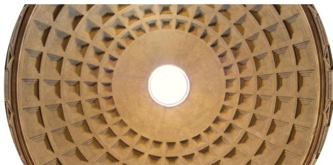
The Pantheon dome - made entirely out of concrete.
