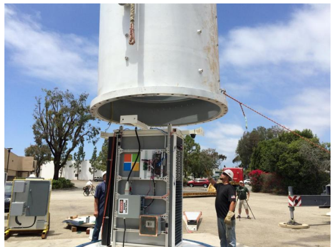
Installing server rack into Project Natick vessel.
