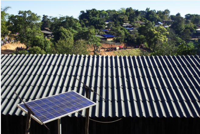
Solar panel on the roof of a house. Credit: Shutterstock / Twonix Studio / WWF
