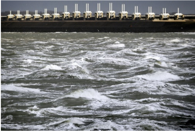
The Eastern Scheldt storm surge barrier (Oosterscheldekering), pictured in Vrouwenpolder, The Netherlands
