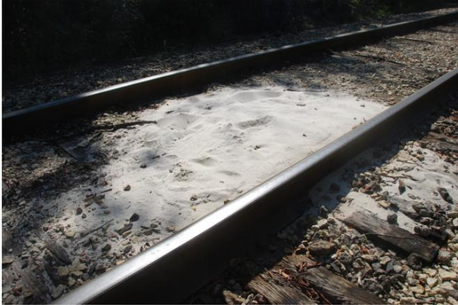
A booming industry in hydraulic fracturing has presented a new challenge: grains of sand can leak from rail cars, accumulate in rail bed ballast and, during a rainstorm, turn into mushy, track-loosening mud. Credit: Tuncer Edil/UW-Madison
