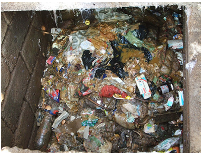
Pit latrines can be filled with solid trash (like this one in
