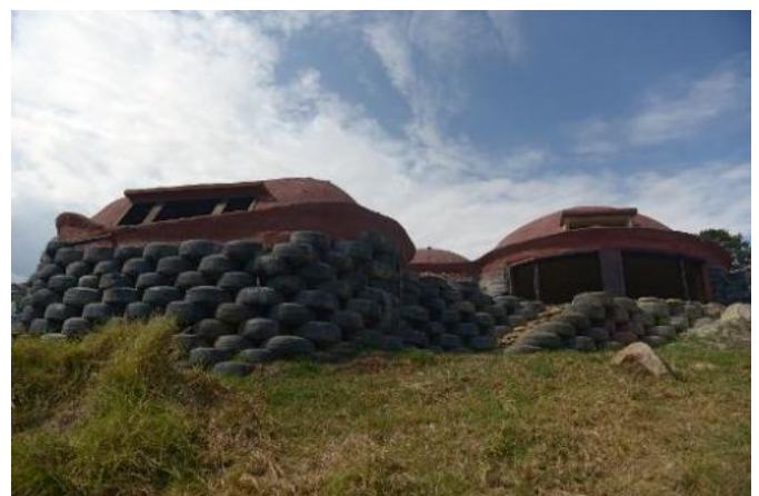
A view of a house built with discarded tires in Choachi, Cundinamarca, Colombia on March 16, 2015
