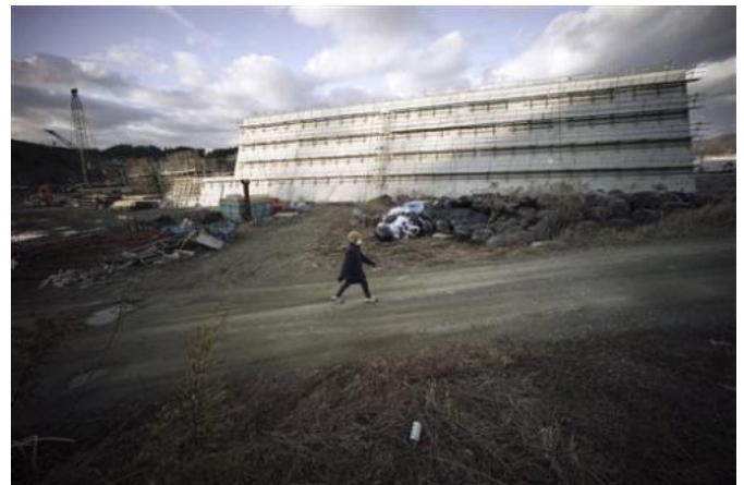
In this March 5, 2015 photo, a woman walks near sea walls being built in Rikuzentakata, Iwate Prefecture, northeastern Japan. Four years after a towering tsunami ravaged much of Japan's northeastern coast, efforts to fend off future disasters are focusing on a nearly 400-kilometer (250 mile) chain of cement sea walls, at places nearly five stories high. (AP Photo/Eugene Hoshiko)
