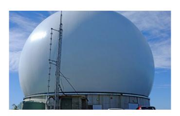
Researchers are using Australian Bureau of Meteorology radars that offer 'dual-polarisation', which allows them to measure hail, or rain, and very accurate rain rates.
