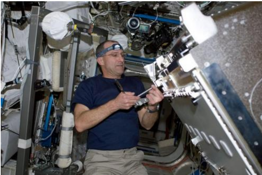
NASA astronaut Don Petit installs the Water Recovery System into the Destiny Lab on the International Space Station in November 2008. Credit: NASA
