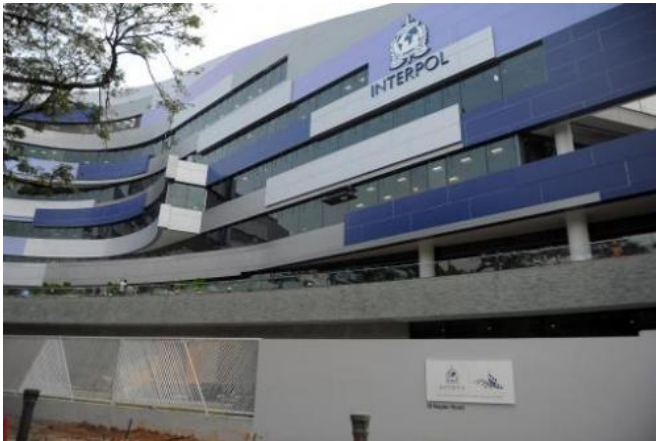
New INTERPOL Global Complex for Innovation (IGCI), pictured in Singapore, on September 30, 2014
