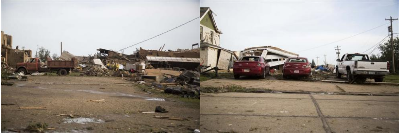
Severely damaged homes and buildings are seen after a tornado on Monday, June 16, 2014, in Pilger, Neb. The National Weather Service said at least two twisters touched down within roughly a mile of each other. (AP Photo/The Journal-Star, Stacie Scott)
