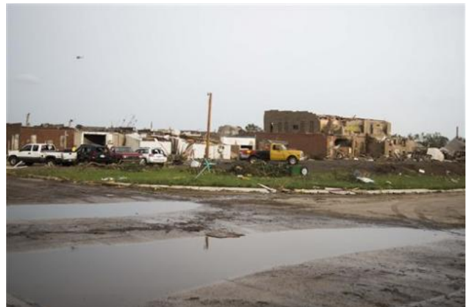
Severely damaged homes and buildings are seen after a tornado on Monday, June 16, 2014, in Pilger, Neb. The National Weather Service said at least two twisters touched down within roughly a mile of each other. (AP Photo/The Journal-Star, Stacie Scott)
