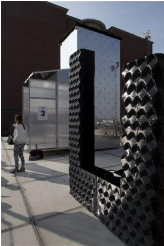
A 3D printer, rear, and part of a printed canal house, foreground, are lit by the sunlight in Amsterdam, Netherlands, Thursday, March 13, 2014. Dutch architecture firm Dus has embarked on a project to build a 21st-century version of a classic Amsterdam canal house, printing it out piece by piece with an oversized 3-D printer, and then slotting them together like oversized Lego blocks. The goal is to discover and share the potential uses of 3-D printing in construction by creating new materials, trying out designs and testing building techniques. (AP Photo/Peter Dejong)
