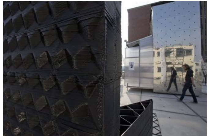
A designer walks over to check the 3D printer, rear, as he passes part of a printed canal house, left, in Amsterdam, Netherlands, Thursday March 13, 2014. Dutch architecture firm Dus has embarked on a project to build a 21st-century version of a classic Amsterdam canal house, printing it out piece by piece with an oversized 3-D printer, and then slotting them together like oversized Lego blocks. The goal is to discover and share the potential uses of 3-D printing in construction by creating new materials, trying out designs and testing building techniques. (AP Photo/Peter Dejong)
