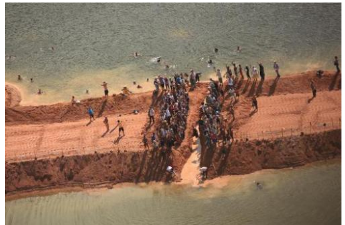
Activists dig a gap through a temporary earthen dam over the Xingu River in Para, northern Brazil, on June 15, 2012 in protest against the massive Belo Monte dam project
