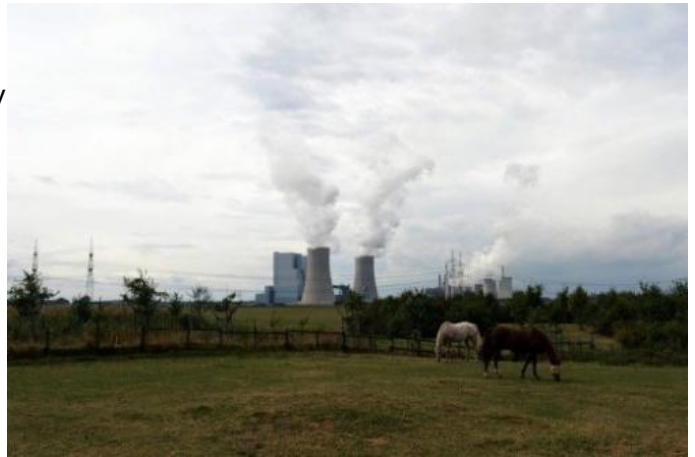
Horses graze in front of the new Neurath lignit coal-fired RWE power station on September 11, 2012 at Grevenbroich. RWE has announced that it will shut down a number of plants—representing combined capacity of 4,300 megawatts—in both Germany and the Netherlands
