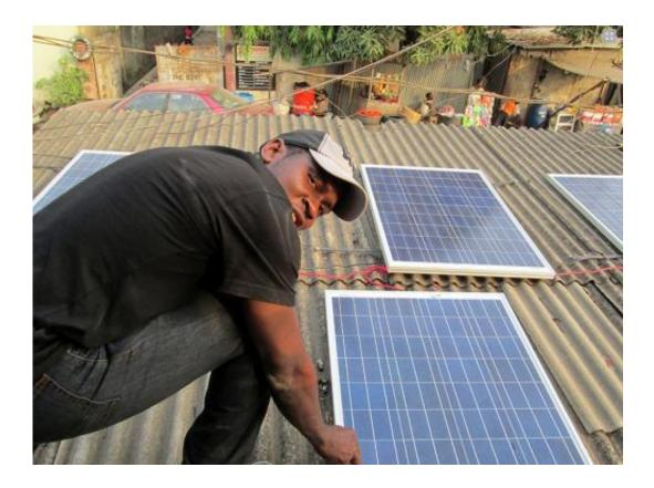
Chidube Ezeozue checks solar panel mountings and connections on a rooftop. Credit: Chidube Ezeozue
