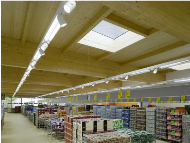
Skylights in the roof reduce power requirements for lighting. Credit: Ralph Kensmann, StartDesign GmbH
