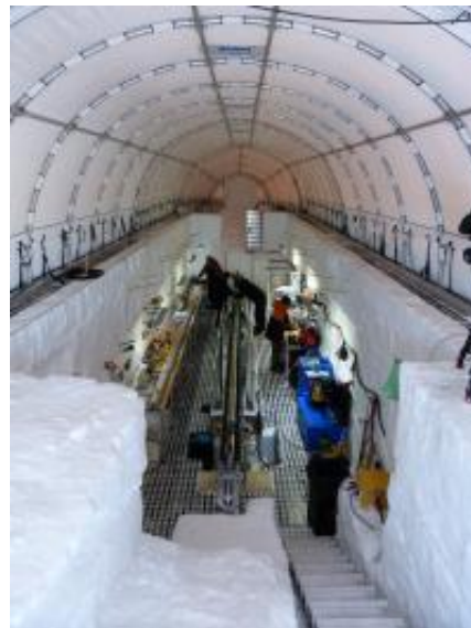
The drill trench tent.
