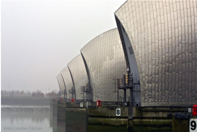
The Thames Barrier was built to protect London from floods with a return period of 1000 years up to 2030. Credit: London-GB.com
