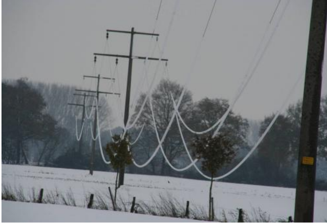
Black ice can be an immense burden on the power grid. The power lines sag low enough to almost touch the ground. Credit: Fraunhofer FIT
