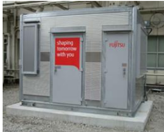
Figure 3: Prototype Container Data Center
