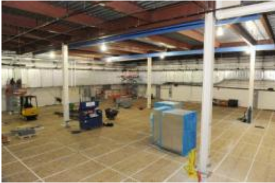
This image shows the MMS cleanroom during construction. Credit: NASA
