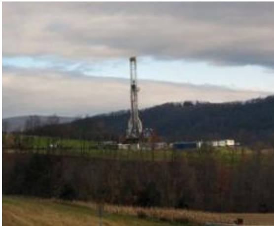
A tower for removing gas at the Marcellus Shale Formation in Pennsylvania. Credit: Ruhrfisch/Wikimedia Commons.
