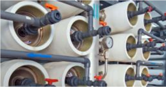
Racks of filters in a desalination plant. Credit: Paul Vinten, through iStockphoto
