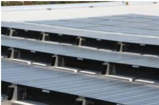
Tilted solar panels (front) create a stronger cooling effect than panels flush with the roof. Credit: Jacobs School of Engineering at UC San Diego
