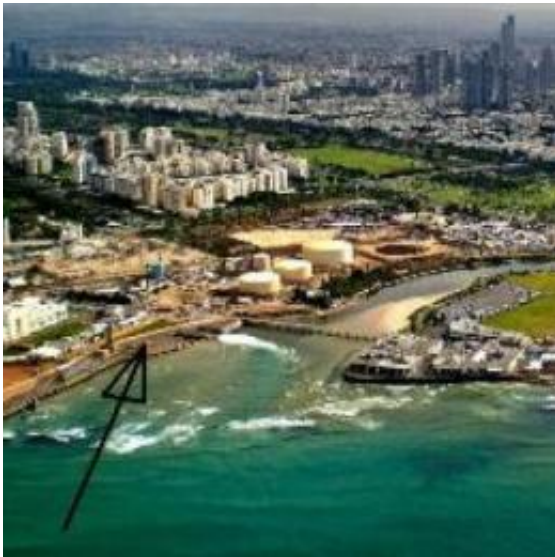
This is an aerial view of the remains of the Tel Qudadi fortress. Credit: Leon Mauldin/AFTAU
