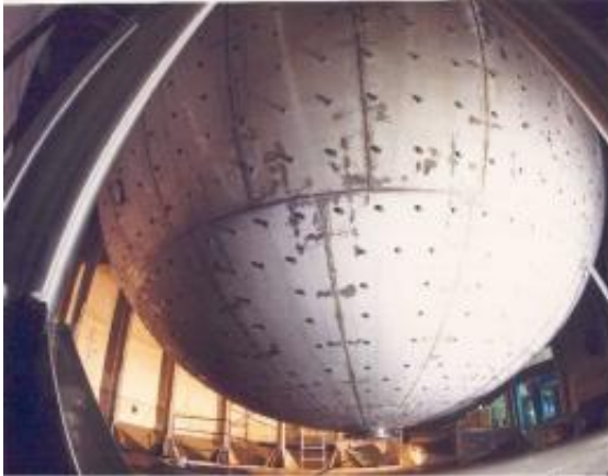
View of the Borexino "Stainless Steel Sphere" (SSS) from from the "Water Tank", before cables and PMTs installation.
