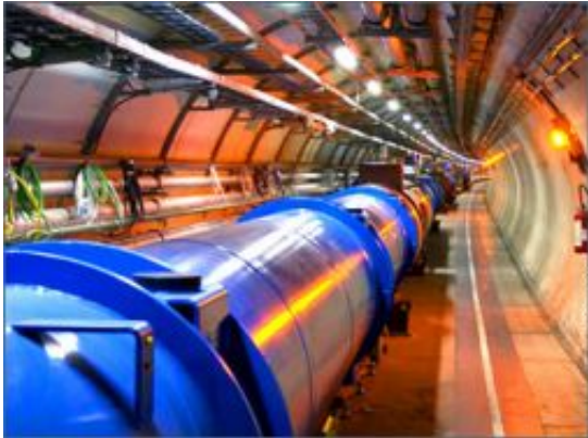
The LHC tunnel
