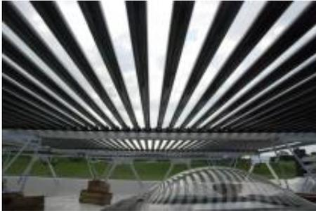
(PhysOrg.com) -- Long cylinders wrapped in a thin dark blue film rest atop a newly constructed home in Central Pennsylvania. Beneath the cylinders is vegetation. The arrangement is not only the engine that powers the house, but may be evidence that the future of solar-powered homes has arrived.
