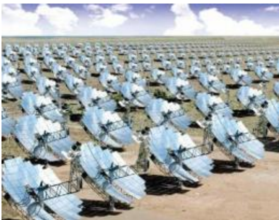
At the Stirling Energy Systems suncatcher dish farm being developed in California, 38-foot-diameter dishes power track the sun and each power a 25 kW Stirling cycle generator. Image credit: Stirling Energy Systems.
