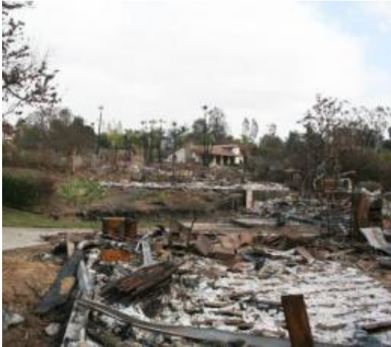
Ruins of two homes in the Trails community burned during the Witch and Guejito fires in 2007. To reduce structure losses from future Wildland Urban Interface fires, NIST has reconstructed a timeline of the fire events, including the defensive actions taken by first responders and homeowners. Credit: Maranghides, NIST
