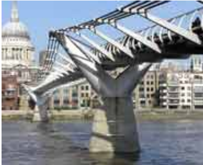
The London Millennium Bridge seen from the south bank of the Thames. Photo by Adrian Pingstone
