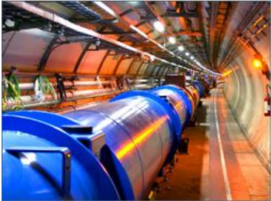
The LHC tunnel
