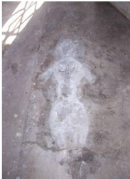
Scientists have determined that this stain on a concrete floor was produced by fatty acids and an acidic cleaner. Photo by: Courtesy of Glen Jackson
