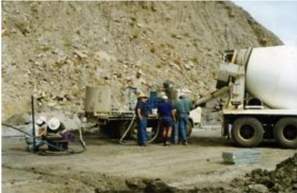
Preparing to cement an experimental geophone string in a borehole in Central Queensland. Image credit – CSIRO
