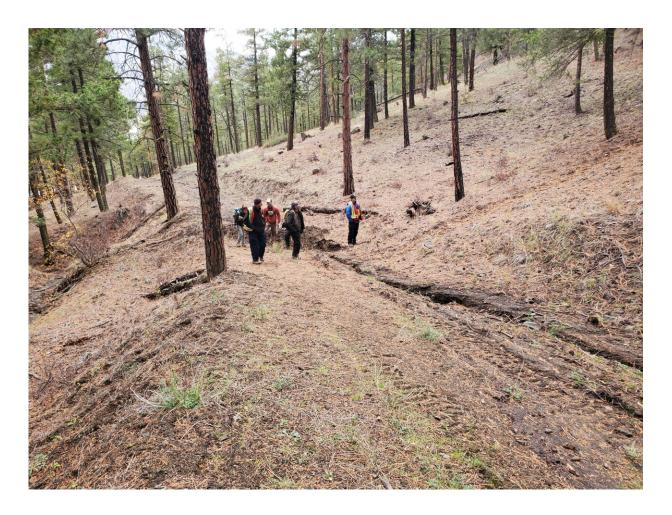
Student Kaushal Gnyawali and Dr. Tannant can be seen standing on top of a one-meter-high deflection berm constructed to protect property on Okanagan Indian Band land. Understanding if the berm is thick enough, high enough and constructed with the right soil material to resist the debris flow forces and volumes are key questions to be answered in the context of climate change. Credit: Kaushal Gnyawali
