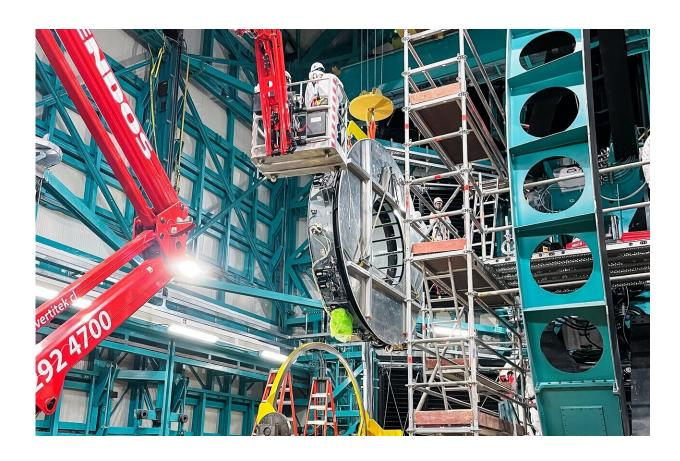
On July 24, 2024, Vera C. Rubin Observatory's 3.5-meter secondary mirror was installed onto the Simonyi Survey Telescope. The installation was successfully completed after installing the mirror onto its support cell and moving the combined structure from Rubin's maintenance floor up to the dome level via the heavy-load platform lift. The secondary mirror is the first piece of glass to be installed into its final position on the telescope. Credit: Rubin Observatory/NSF/AURA/S. MacBride
