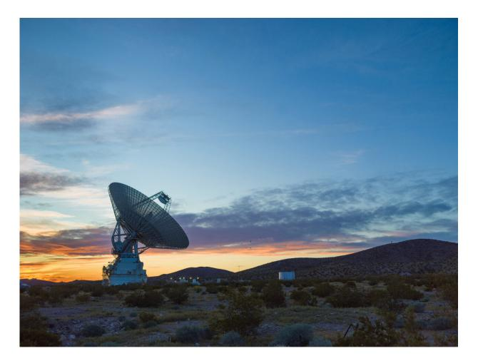
This sunset photo shows NASA's Deep Space Station 14 (DSS-14), the 230-footwide (70-meter) antenna at the Goldstone Deep Space Communications Complex near Barstow, California. NASA/JPL-Caltech
