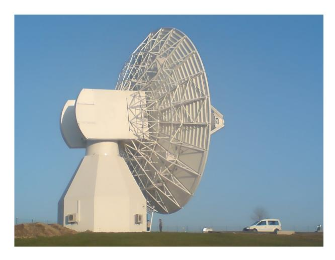
The LEGS antennas (similar in appearance to this 20.2-meter CPI Satcom antenna) will be placed in equidistant locations across the globe. This ensures that when the moon is setting at one station, it will be rising into another's view. With the moon constantly in sight, NASA's Near Space Network will be able to support approximately 24/7 operations with moon-based missions. Credit: CPI Satcom
