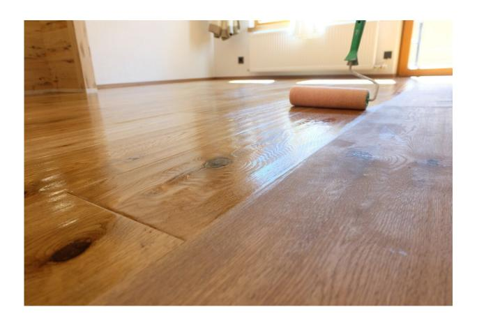
Without a coating, UV light can interact with wood surfaces, causing discoloration and damage. Credit: Naturhaus Naturfarben GmbH
