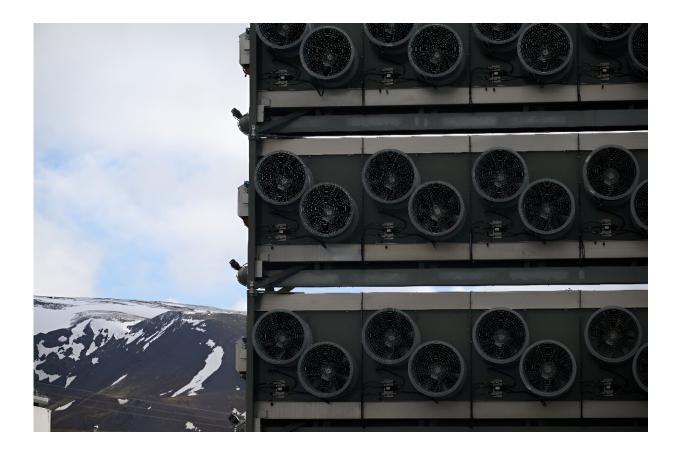
A nearby geothermal energy plant powers Mammoth's fans and heated chemical filters that extract CO2.
