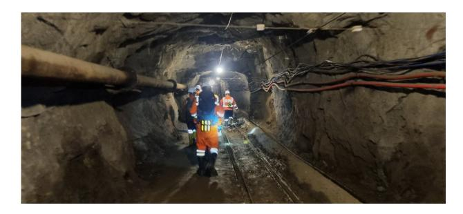
The team of scientists exploring the mine galleries under the guidance of local miners. The team of scientists monitoring hydrogen concentration in the air of a mine gallery, and sampling gas seeping in the water draining stream. This gallery is located 1,000 m below the surface. Credit: F-V. Donzé
