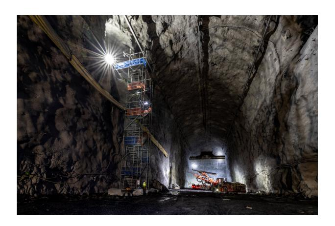
Construction workers created two colossal caverns, each more than 500 feet long and about seven stories tall, for the gigantic particle detector modules of the Deep Underground Neutrino Experiment, hosted by Fermilab. A third cavern will house utilities for the operation of the detector. Credit: Matthew Kapust, Sanford Underground Research Facility
