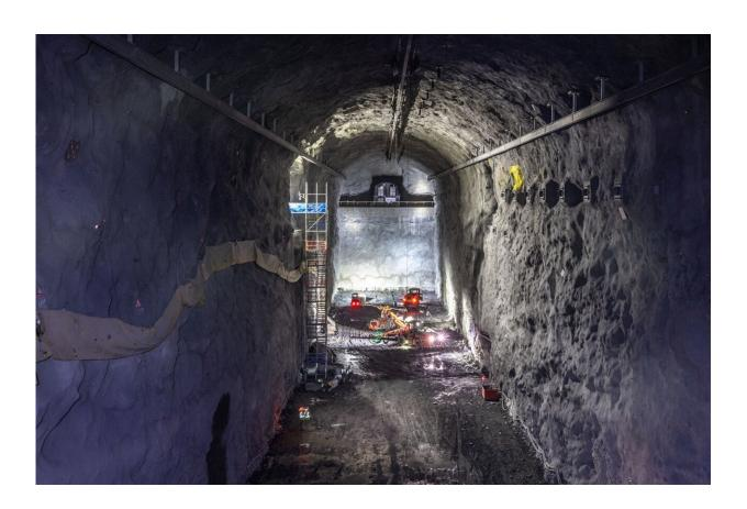
A bird's eye view of one of the large caverns in South Dakota, about the height of a seven-story building. Large particle detectors for the Deep Underground Neutrino Experiment will be placed here to study the behavior of neutrinos. The DUNE detectors are expected to be the largest underground cryogenic system in
