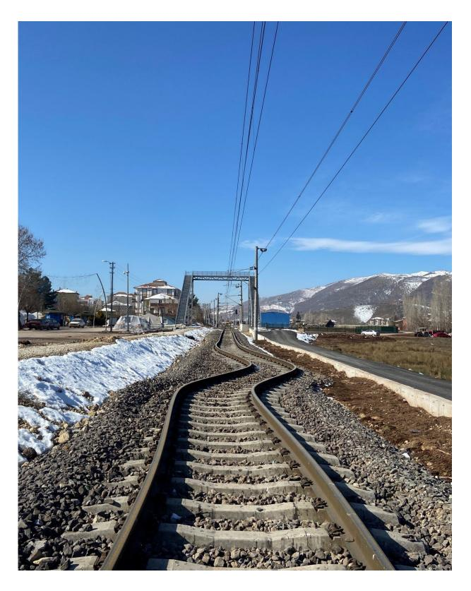
Strongly deformed railway track after the 2023 Turkey earthquake sequence, resulting from both ground shaking and liquefaction. The railway track has been
