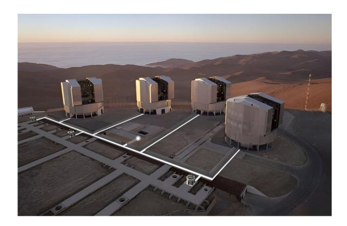
This aerial view shows the ESO's VLTI, the Very Large Telescope Interferometer. It has a total of eight separate, movable telescopes that can all look at the same object, increasing the interferometer's angular resolution. Credit: ESO
