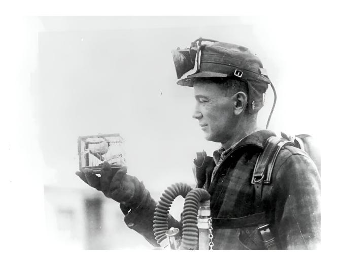
Mining foreman R. Thornburg shows a small cage with a canary used for testing carbon monoxide gas in 1928. Credit: George McCaa, U.S. Bureau of Mines
