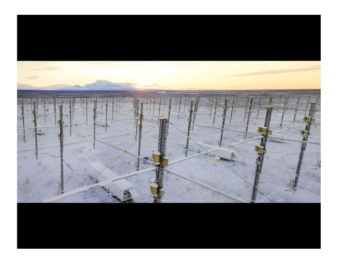
HAARP's Ionospheric Research Instrument is a phased array of 180 high-frequency antennas spread across 33 acres. Credit: UAF/GI photo by JR Ancheta.
