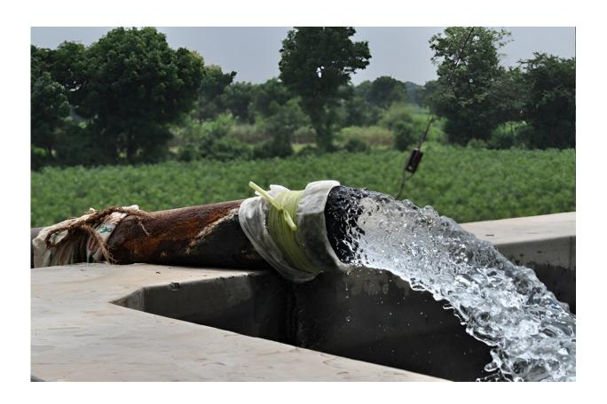
A bore well pumping groundwater to irrigate fields in Gujarat, India. Wells in this region can pull groundwater from up to 800 feet below ground, and water tables are falling rapidly due to overexploitation. Credit: Meha Jain, University of Michigan.
