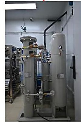
Air PSA separation equipment with production rate of 5 Nm 3 /h-N 2
