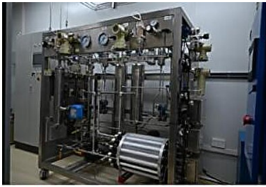
Alkaline water electrolysis equipment with production rate of 3 Nm 3 /h-H 2
