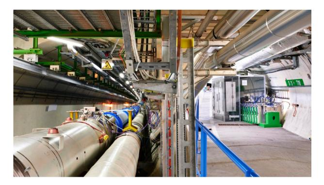
A section of CERN's Large Hadron Collider (left) and the new experiment SND@LHC (right). Neutrinos are produced at one of the LHC's collision points, hidden behind the curvature of the accelerator, and interact in the SND@LHC detector after traversing around 100 meters of rock and concrete. Credit: Brice, Maximilien; SND@LHC Collaboration.
